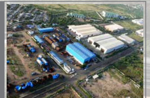
KANDLA SEZ WORKS
